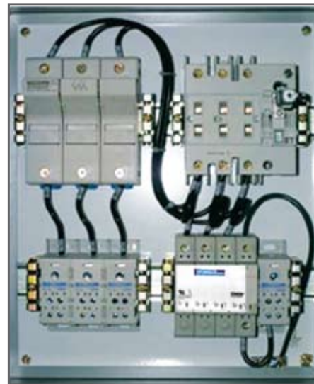
Surge-Trap applied in an electrical panel.
